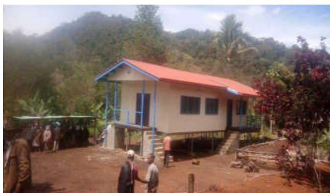
Figure 45 Kuga (Paikone) Village Court House in WHP.
