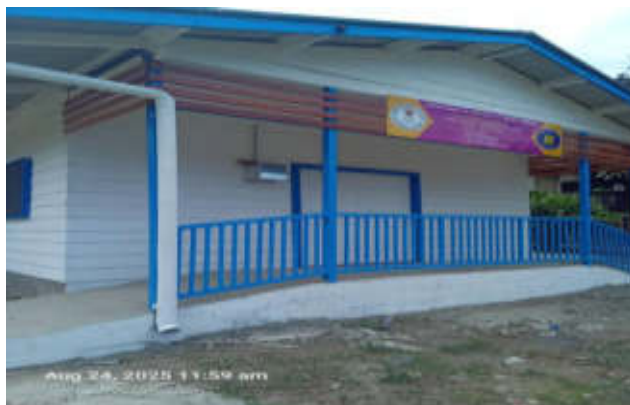
Figure 43 Paril Village Court House in NCD (Motu Koita).
