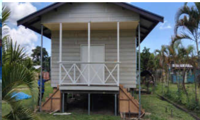
Figure 44 Bitapaka Village Court House in ENB.
